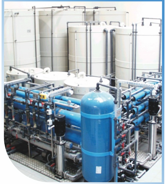
Purification and recycling of waste water from the manufacture of aircraft parts with ZLD technology. GE Aviation Hungary Ltd. / Hungary 100 m 3 /day
